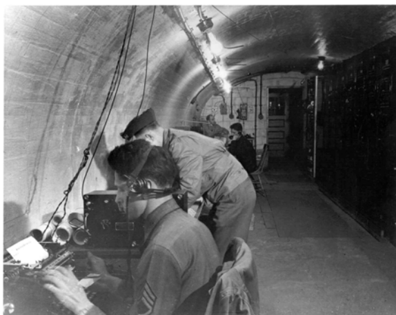
Switchboard Room, HDCP, Ft. Hancock
