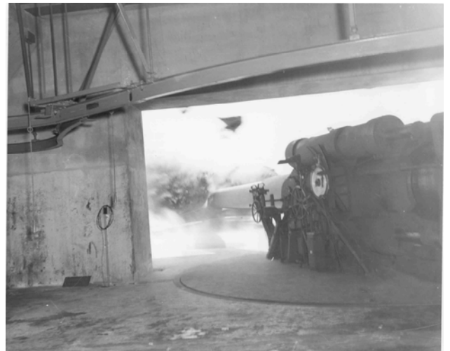
Battery Kingman casemate firing 1943
