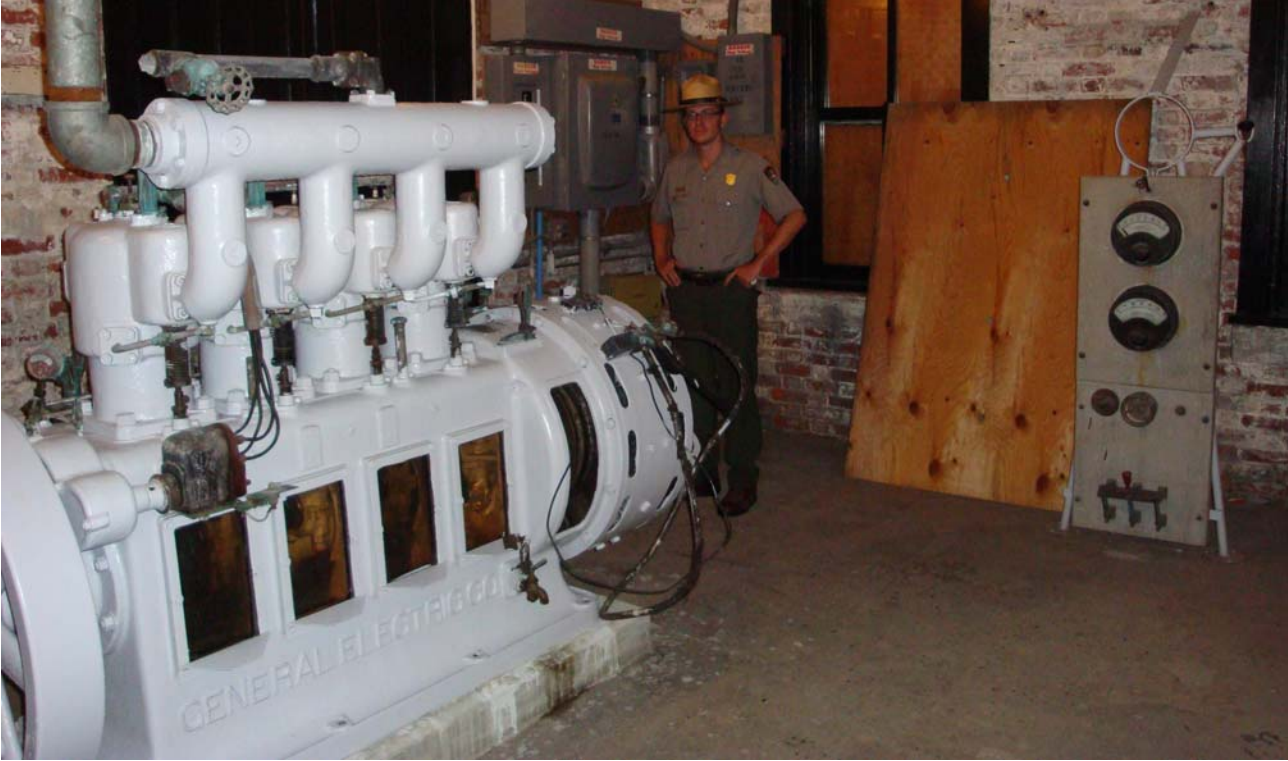
A close-up of the 25kw generator and its radiator is below. Glass panels allow viewing of the crank shaft.
