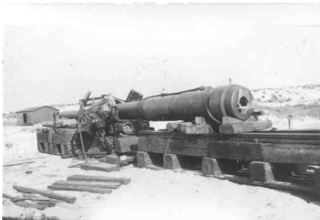
Assembling 6-inch M1900 rifle
