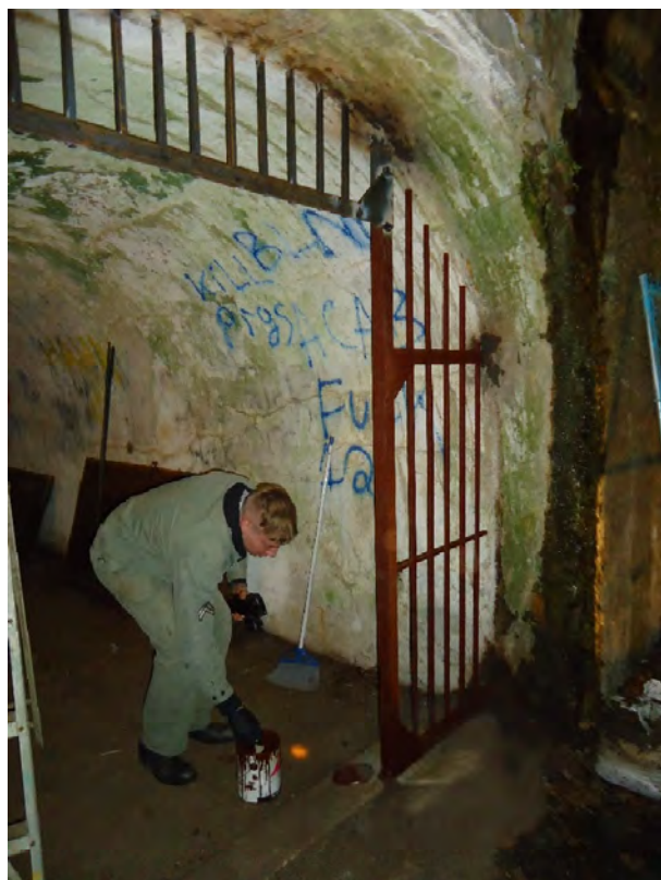
Below CPL Bujdos is finishing the priming of the left-side frame.
