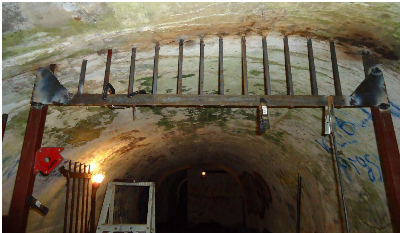
Below CPL Bujdos is finishing the priming of the left-side frame.
