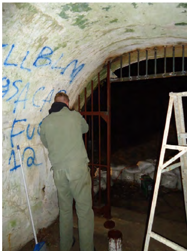
Below CPL Bujdos is finishing the priming of the left-side frame.
