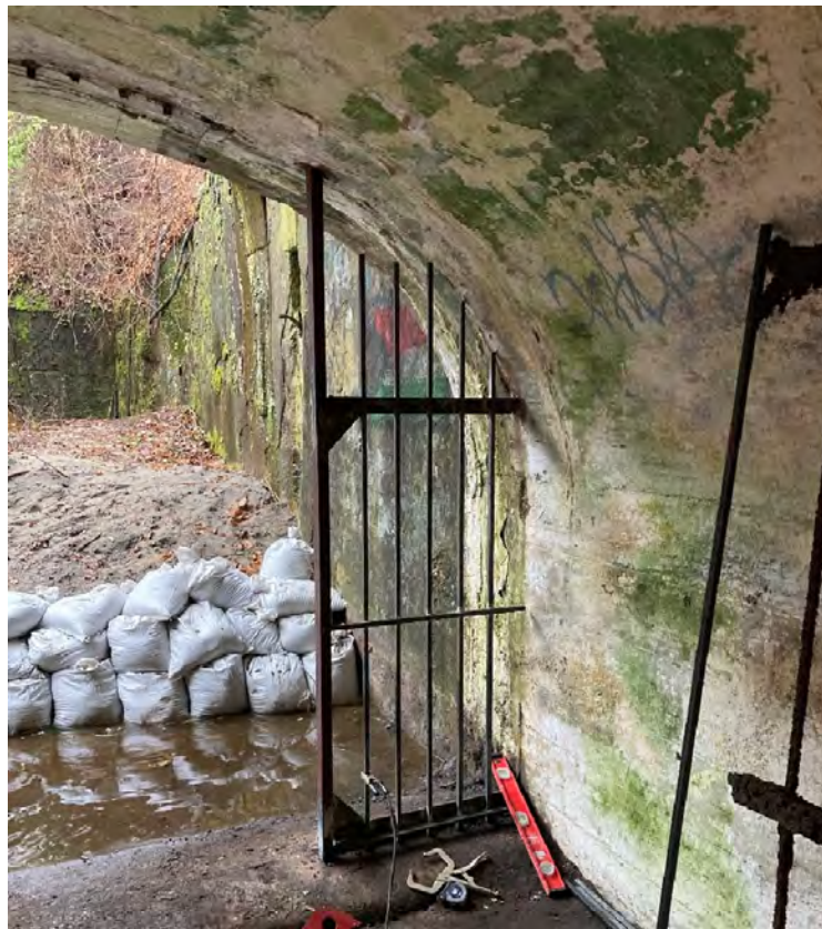
Below is the first section of the frame welded into place in March 2024.
