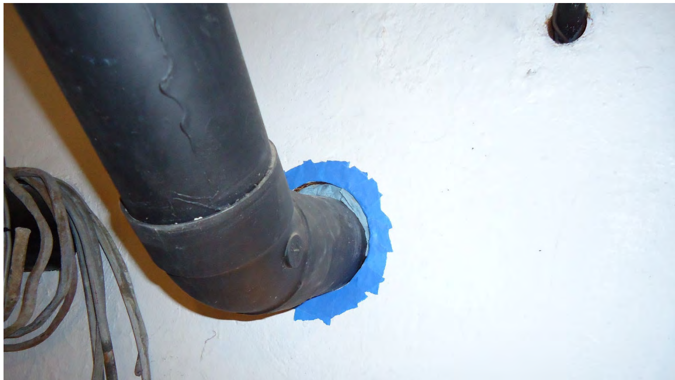
A closeup photo of the caulking action inside the plotting room before application of the black caulking material.
