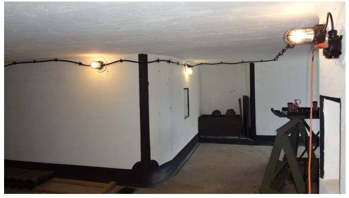
The view below shows the completed lighting inside the powder passage. Only a few cable hangers remain to be restored and installed. This is the lighting installation much as it looked from the late 1910s to the 1940s. The large racks on the right side of the wall are for gun implements such as ram-rods and cleaning staffs.
