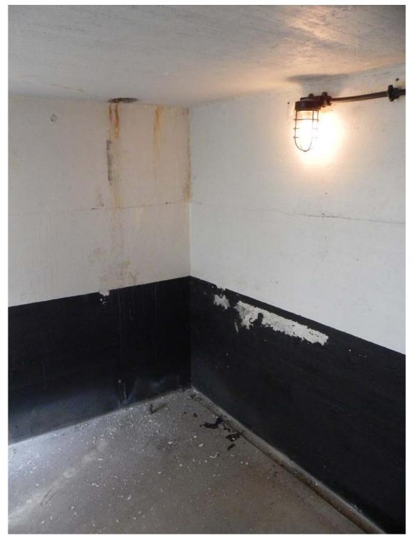
The photo below shows the results of running a paint knife across the wall...the paint just flaked off.
