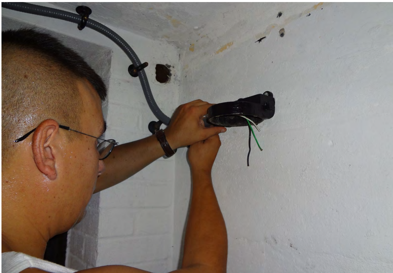
Below the COE Standard Wall light is being installed in the Chemical Decontamination chamber.
