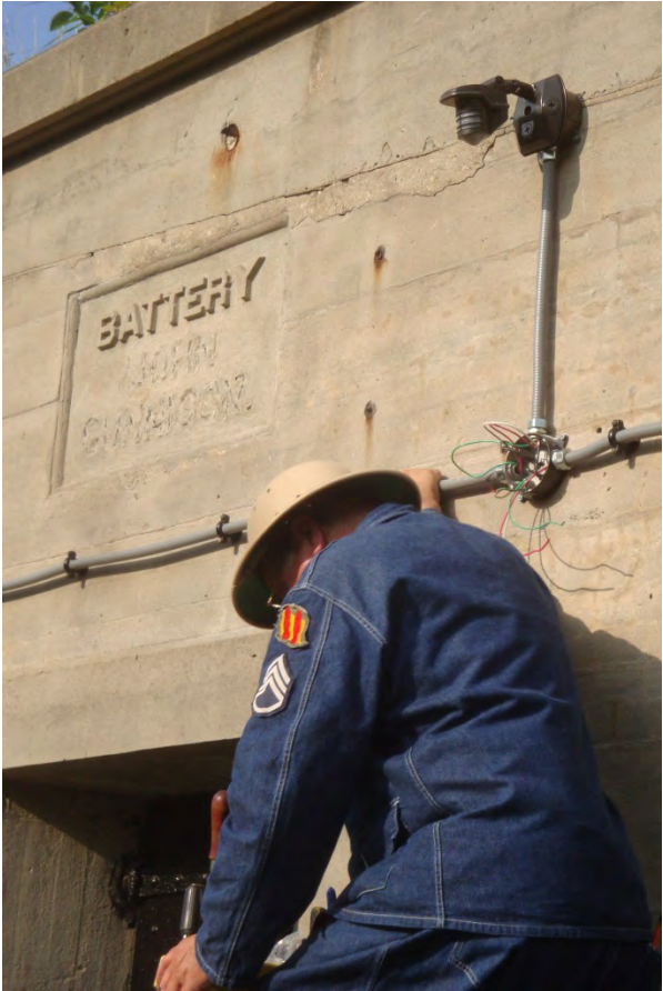
The two photos below show completion of a modern wall light on Gun #1 side (left) and the final installation of the sensor switch (right).
