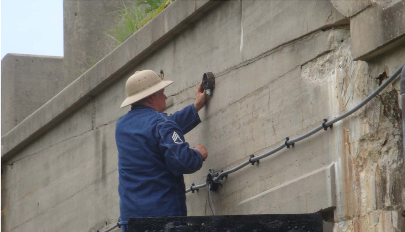
In the photo below the sensor box is being installed.
