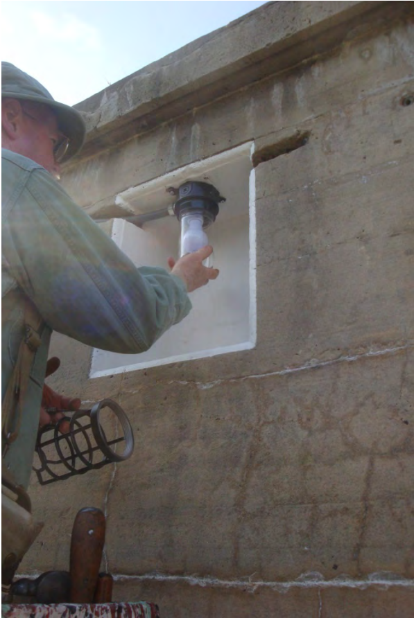
The two photos below show completion of a modern wall light on Gun #1 side (left) and the final installation of the sensor switch (right).
