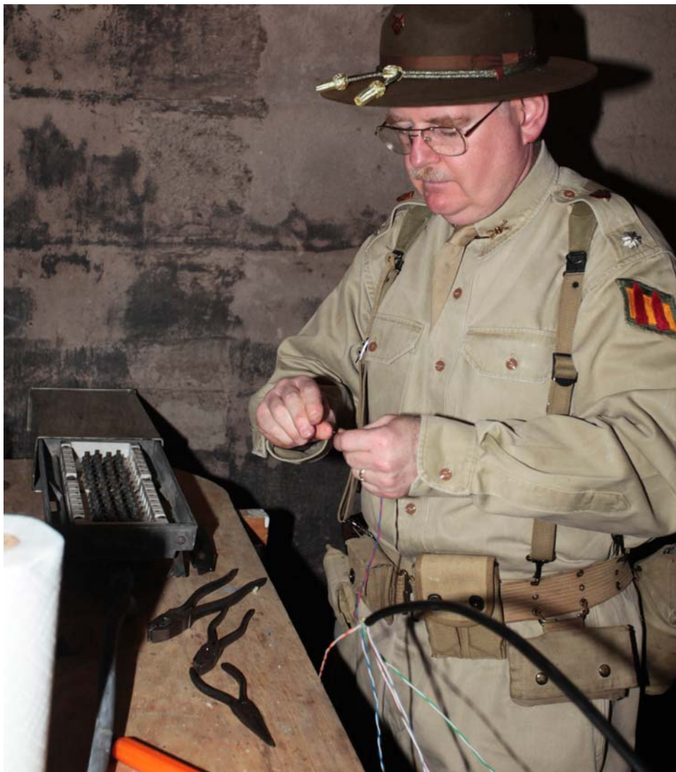
The photo below shows the 6-pair cable as it terminates in the Battery Arnold Commander's Station.
