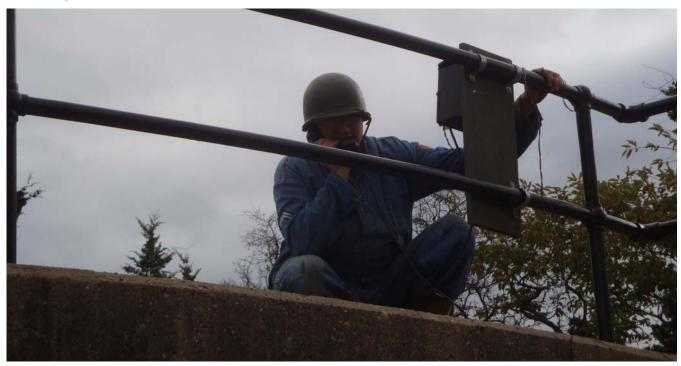
As CPL Meiselman installed telephones, PVT Schafer installed the two gun platform lights. These fully-restored circa 1915 lights are the only known working examples of their kind in the country. Then and now, these lights provide illumination for the Coast Artillery gun crews during night time hours, and were showcased to the public during the Lantern Tour.
