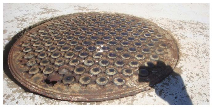
The photo below shows the glass light inserts from the inside of the cable hut. This is a unique and effective way to provide lighting inside the cable hut to enable the Signal Corps personnel to work on the telephone wires without requiring additional lighting.
