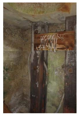
Typical of the early 1920s fire control cable huts, the top has a "glass light magnifying" panel. This is an extremely effective natural lighting technique, dating back to the age of sail. The exterior of the glass magnifiers are shown below.
