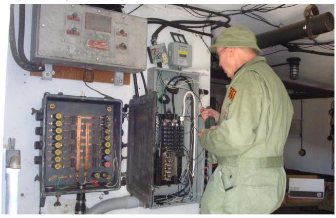
In the photo below, T-5 Komorowski, LTC Welch, and PVT Kaiserman are pulling cable through the conduit to enable controlling of lights in the tool room, chemical warfare room and the magazine from the Corps of Engineers panel box. Completion during this event marked a major milestone in the ongoing restoration of the Battery.
