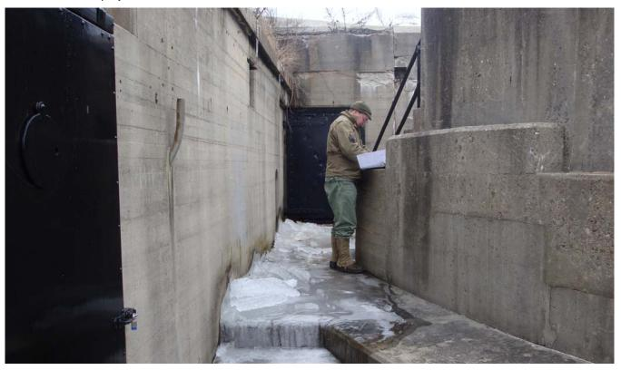
The amount of ice at the battery is apparent in the photo of SSG Weaver below. One of AGFA's goals is to refurbish the original concrete gutter drainage system at the battery, thereby preventing such dangerous overflows and buildups of ice on level surfaces.
