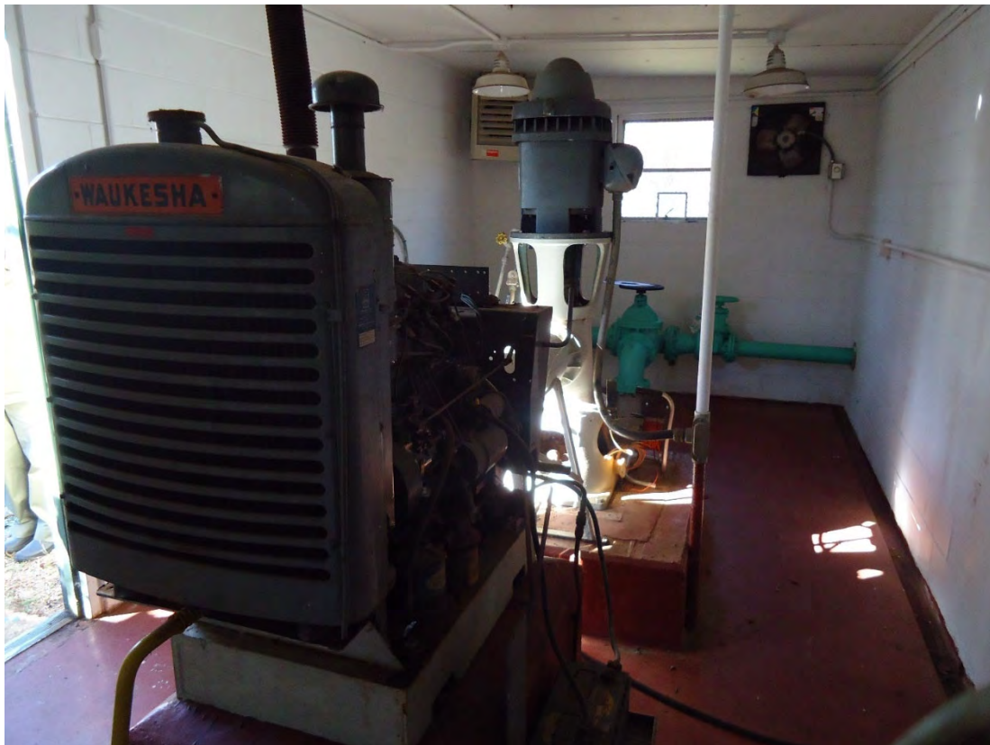
The pump backup gasoline motor is present in the foreground.
