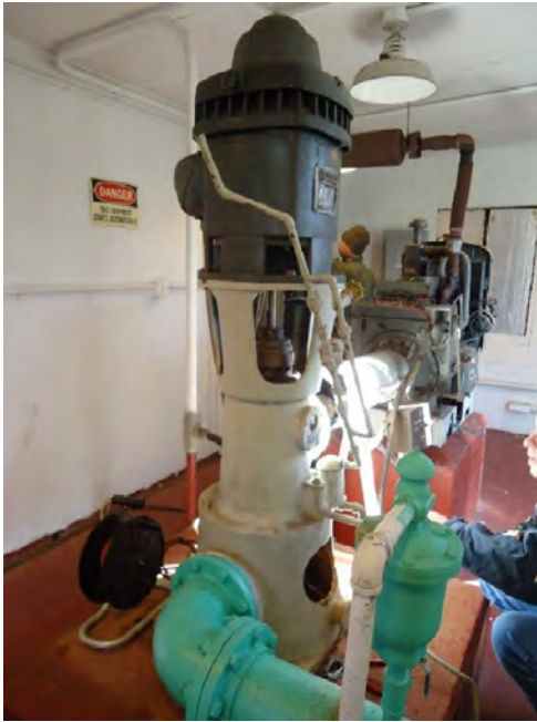
The pump backup gasoline motor is present in the foreground.
