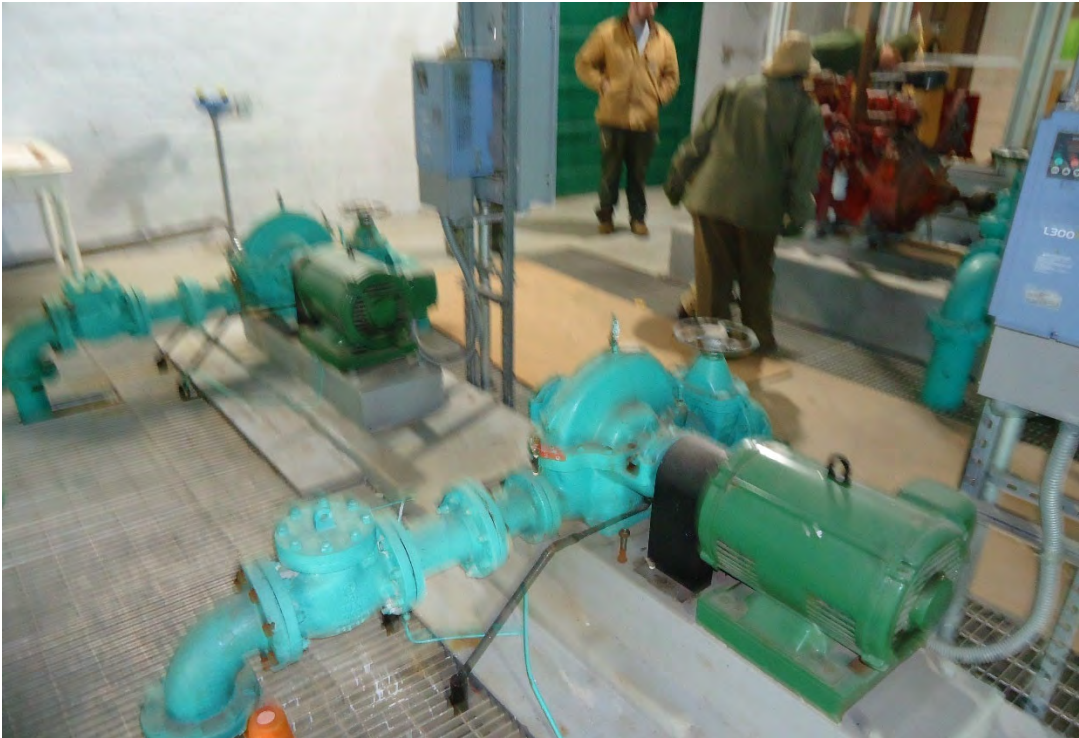
The two pumps below are the main source of water movement in the filtration system.
